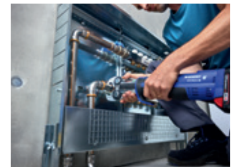
Proven billions of times over: Geberit Mapress Therm works just like any other Mapress system. No new tools are required.
