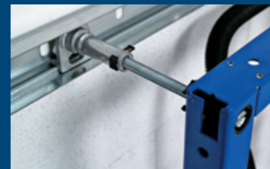
↑ Place the Geberit Duofix installation element in the correct position. For part-height prewalls, fasten with a wall anchor...
