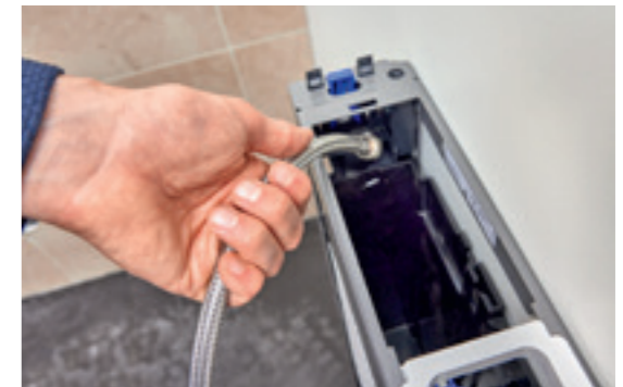
↑ The reinforced braided hose for the water supply connection can be built in without having to remove the flush water tank – that's one less step.
