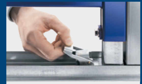
↑ ... and then secure using Geberit Duofix system rail clips.
