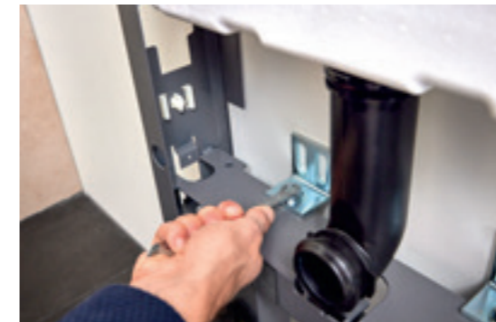
↑ Tried-and-tested mounting brackets are used to fasten the frame to the building structure.
